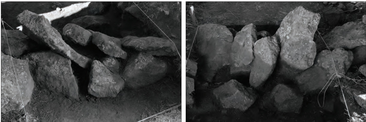
Figure 2.14. Photographs showing the foundation of Enclosure 4. Right: exterior; left: interior.
